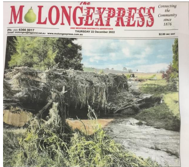
Plate B5.18 – Extract of Molong Express showing build-up of debris on upstream side of Molong Creek Railway Bridge.
