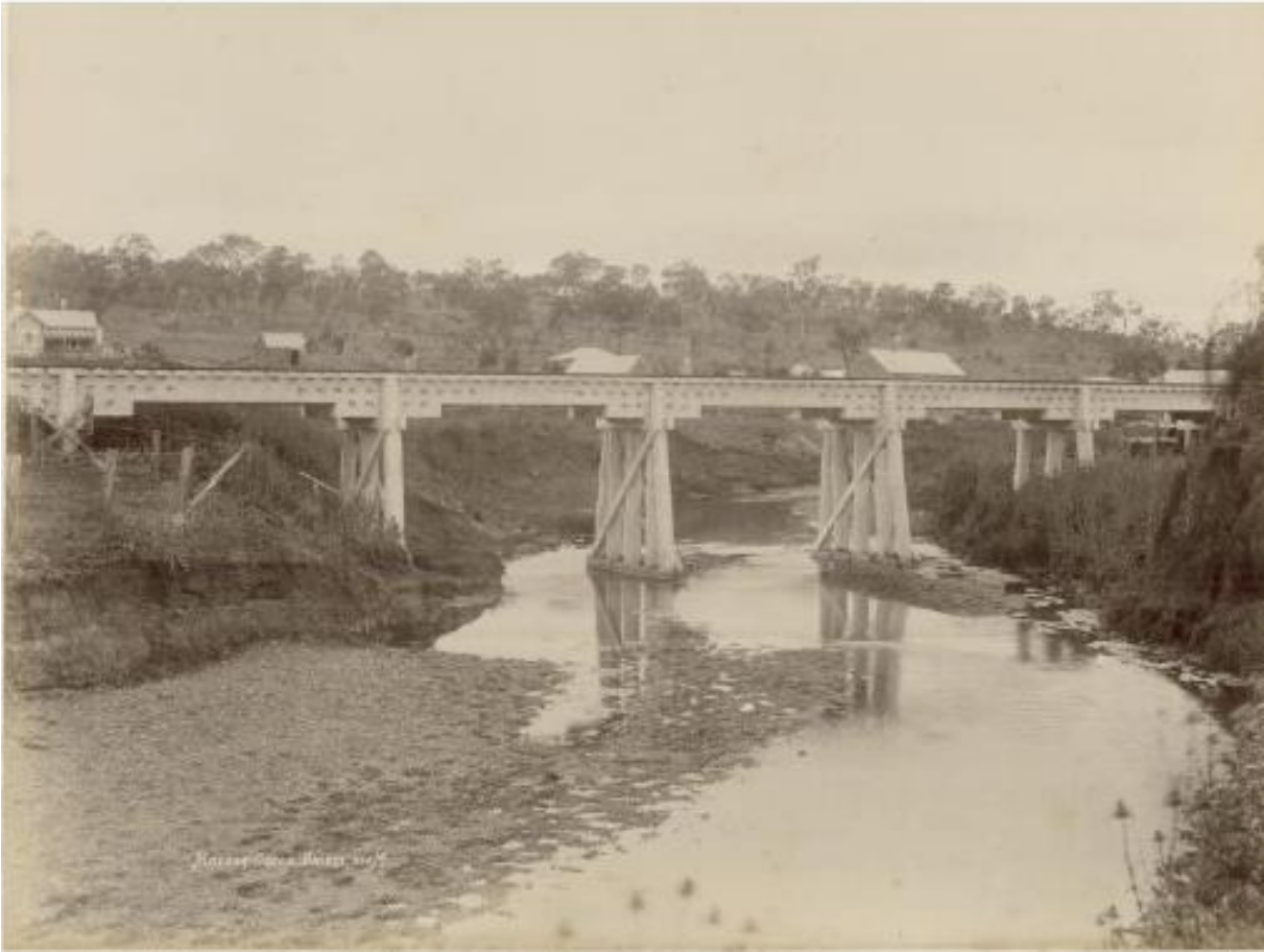
Plate B6.1 – Old Molong Creek Railway Bridge crossing of Molong Creek.
