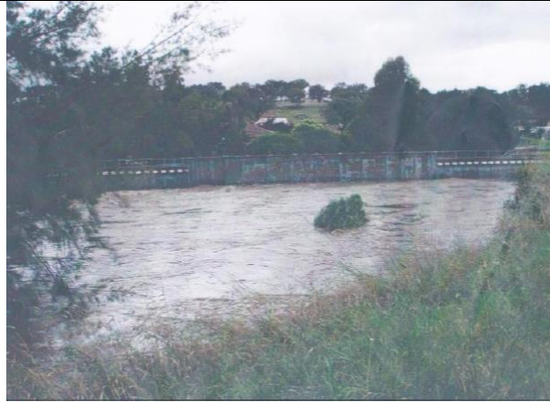
Plate B1.1 – (unknown time) Upstream side of Molong Creek Railway Bridge.
