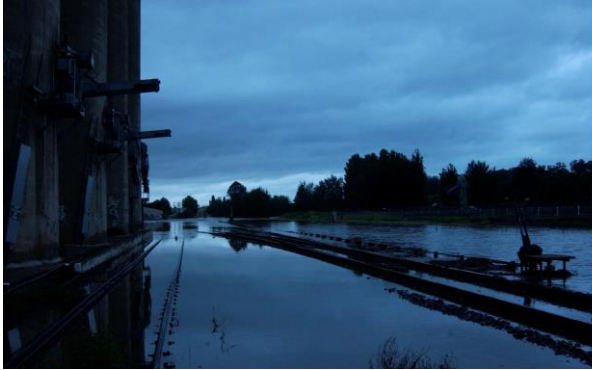
Plate B1.6 – (unknown time) Looking north along Railway adjacent to grain silos.
